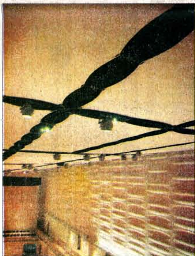
INSIDE THE concert hall, fabric is stretched across the ceiling. It can be used to "tune" the hall, adjusting to control and change the quality of sound.
